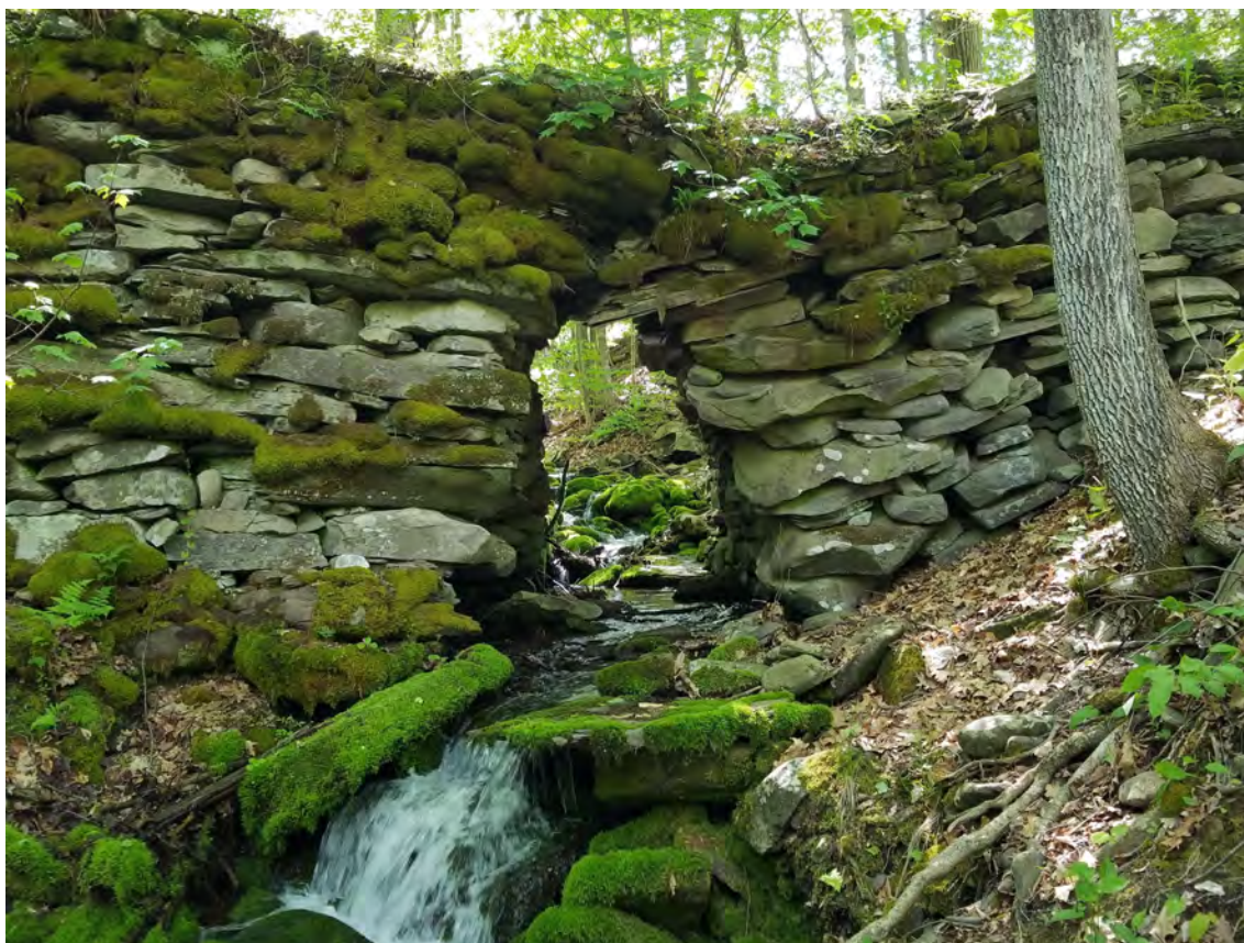
Stone bridge along Giggle Hollow Trail. Photo by Jason Pelton #3013 W1211
