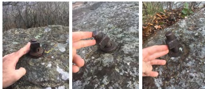
Bolt, nut, and washer assembly on the summit rock of High Point, arranged in a triangle, which would have held down the wooden legs of the signal station tripod for the U.S. Coast and Geodetic Survey.
