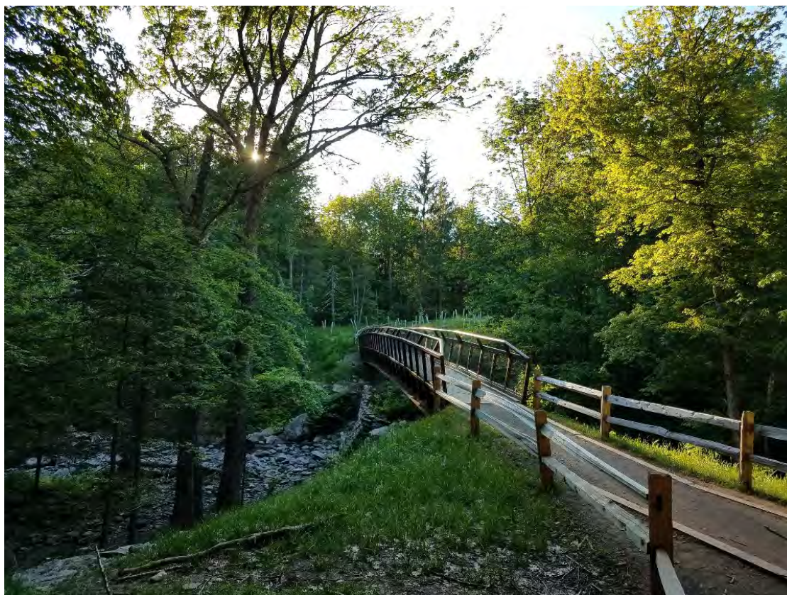
The bridge above the Kaaterskill Falls Photo by Sara Gulbrandsen, #2376 W956
