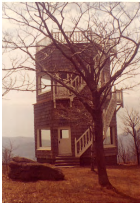
Glen Tonche Tower 02. Courtesy of Bryn Athyn Historic District Archives at Glencairn Museum. Photograph ID: RMP_GT_0106.
