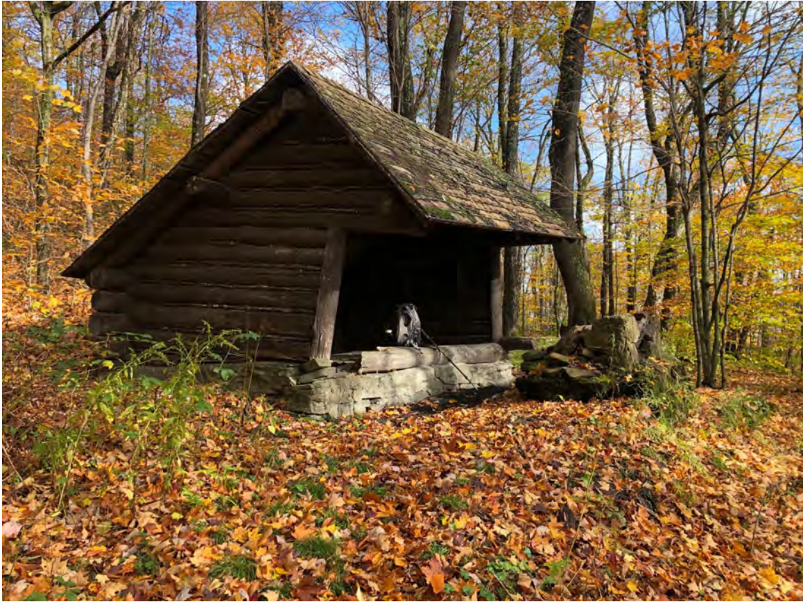
Belleayre lean-to. Photo by Ralph Ryndak #1186 W451
